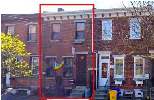
Jasper St house ready for rehab
