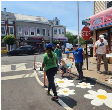
East Trenton EXPO Project Bump Out Installation and Paint Day.
