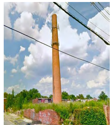
Site of former Croft Mills factory, corner of Broadway & Jefferson
