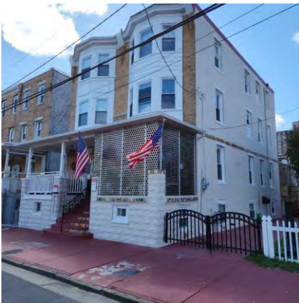
Residential Rehabilitation and Facades
