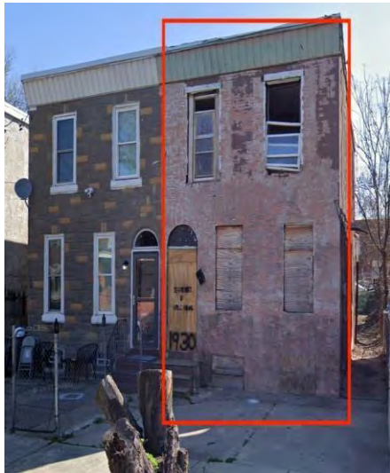
Example of vacant house on Filmore St
