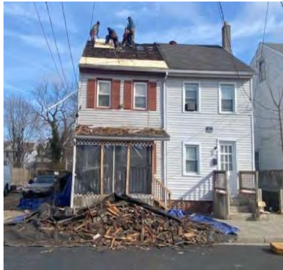
Recently completed home repair project
